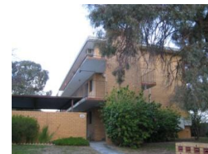
3/28 Carrington St Inglewood
