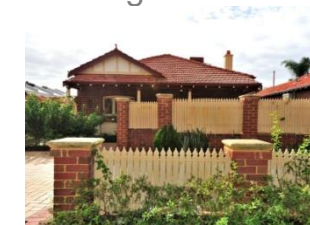
208 Crawford Road Inglewood
