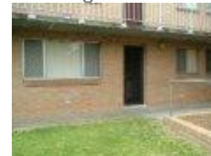
7/38 Carrington St Inglewood
