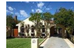
343 Crawford Road Inglewood
